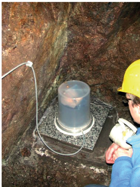
Figure 3.5: The FGE fluxgate magnetometer installed in the mine. Through the transparent plastic cover the sensor and a bag full of orange colored desiccant can be seen.
